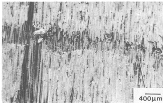
Figure 16 Erosion of the surface of the GRP rod by electrical activity (shedding has been removed).
